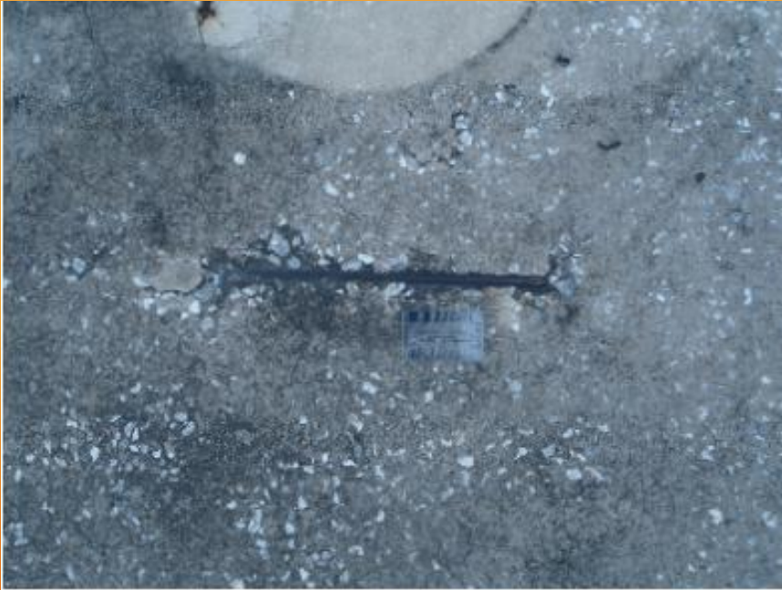
Photograph 20: Corroded bent plate bearing Seats and embeds
