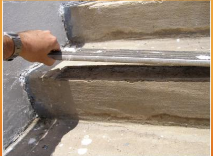
Photograph 23: Loose stair tread nosing
