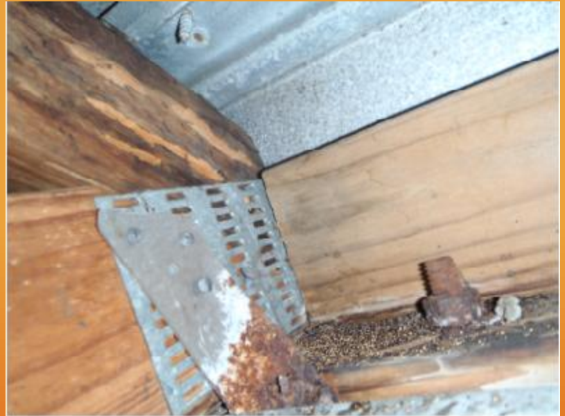
Photograph 38: Damage to roof framing and Connections
