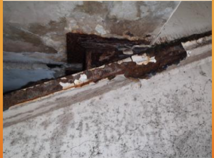
Photograph 20: Corroded bent plate bearing Seats and embeds
