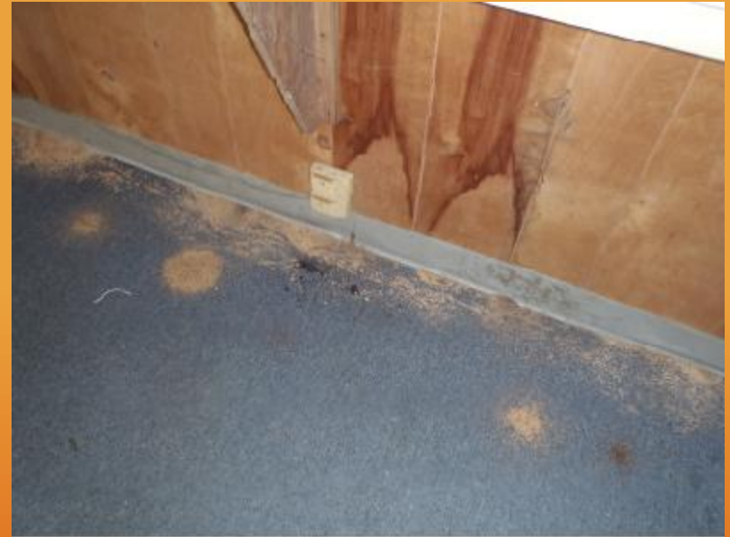
Photograph 43: Appears to be termite frass On floor
