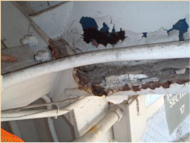
Photograph 2: Closer View of high eave truss connection showing corrosion and section loss
