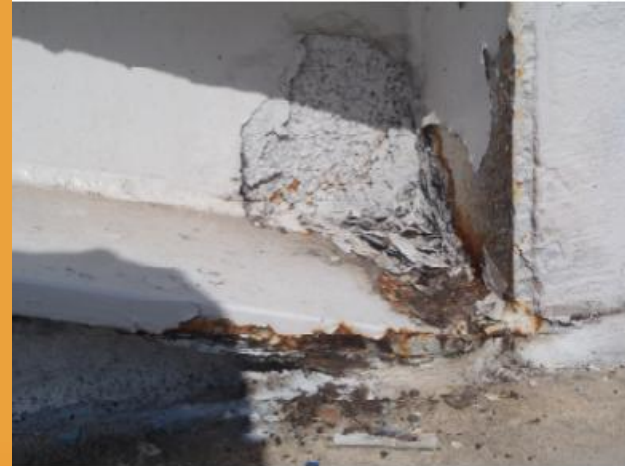
Photograph 8: Corrosion and section loss at raker bearing
