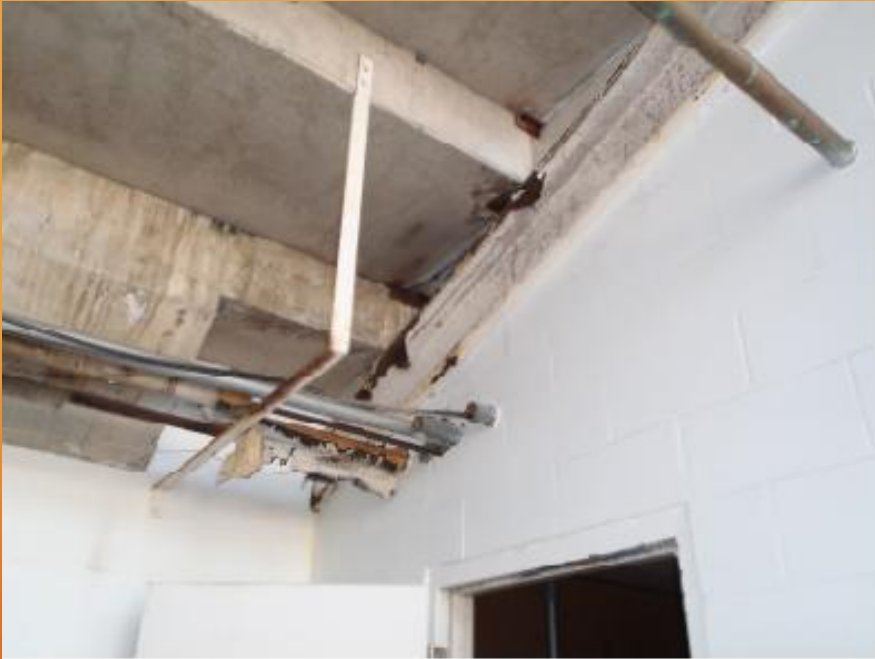
Photograph 19: Seating riser bearing on raker
