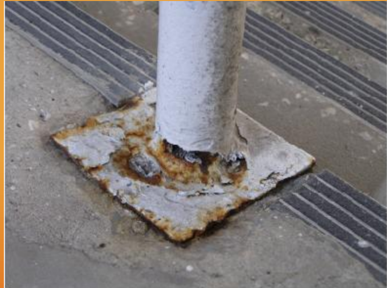
Photograph 27: Corrosion of handrail post Base plate
