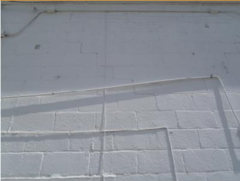
Photograph 41: Stair-step cracks in south wall Of press box building
