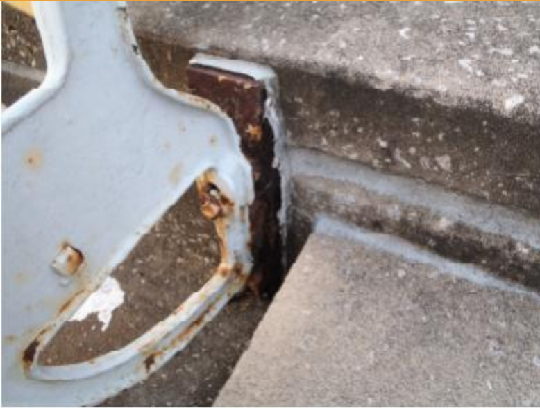
Photograph 26: Failed sealant around seat Anchorage plate
