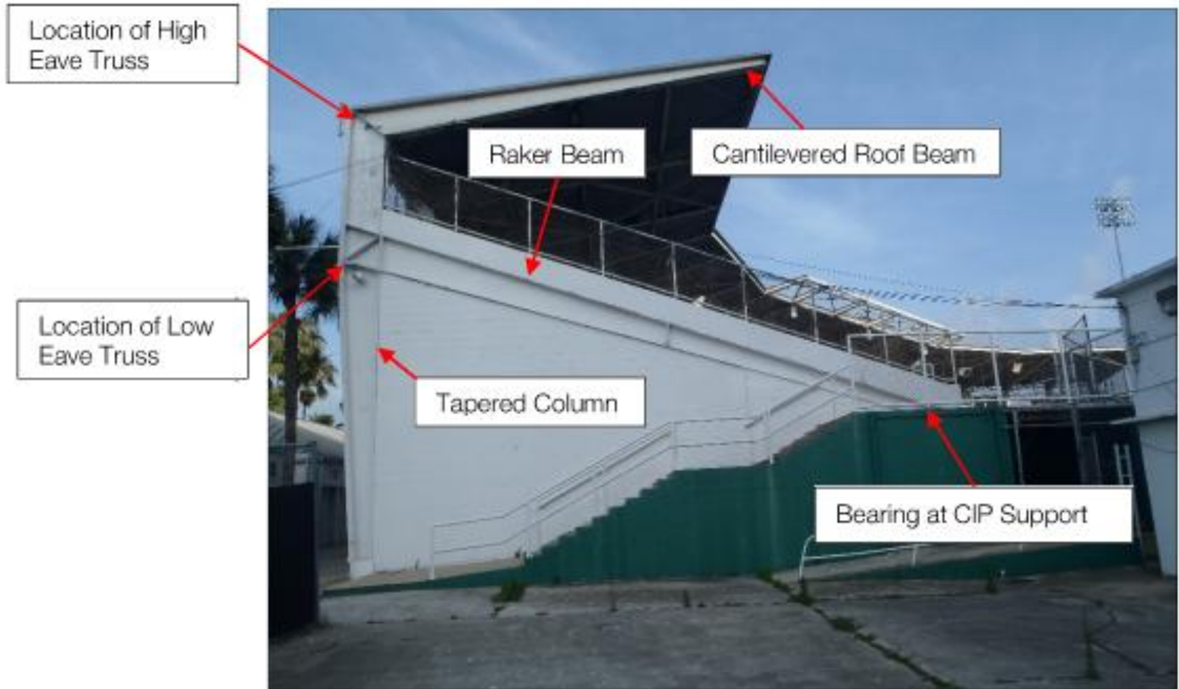
Figure 5: View of existing rigid frame bent.
