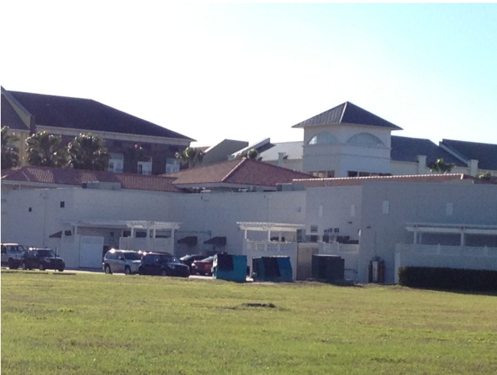
View of the existing commercial building service area adjacent to Lot 629.
