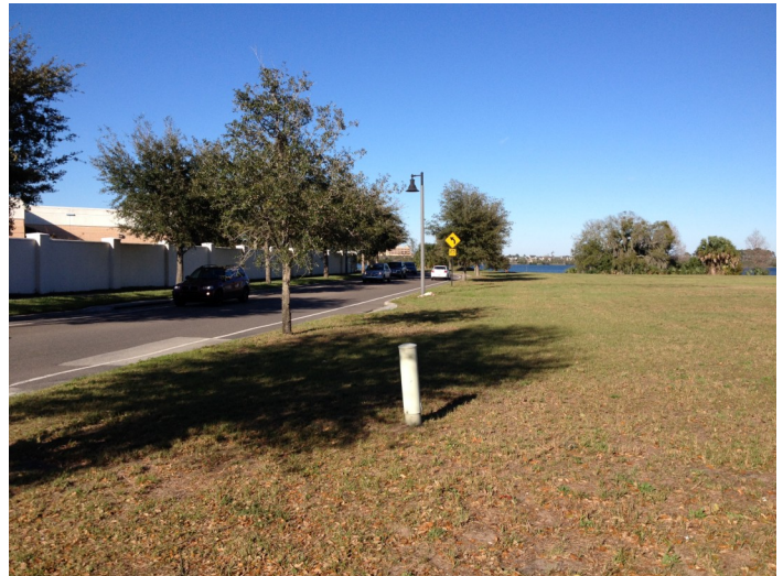
View of Lakemont Avenue, where new on-street parking is proposed within the right-of-way.
