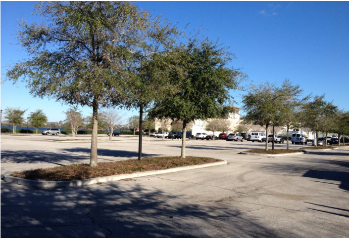
View of the existing temporary parking lot (240 spaces) on Lot 626.
