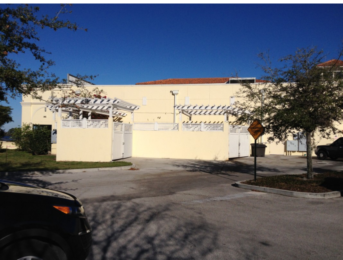
View of existing commercial building service area and dumpster enclosure.
