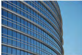
G5 - LAMINATED GLASS WITH CERAMIC FRIT BOD - VIRACON CLEAR GLASS WITH HIGH- OPACITY WHITE SILK-SCREEN #5006 1/8" DOTS
