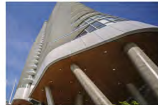
STN1 - NATURAL STONE BOD - COLDSRING - SIERRA WHITE GRANITE - HONED
