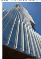
M1 - COATED ALUMINUM EXTRUSIONS BOD - KYNAR SILVERSMITH
